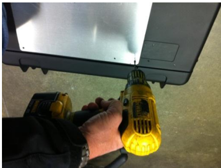
Use holes on plate as drilling template
